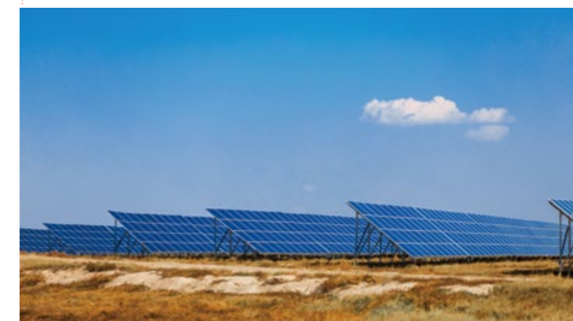
Photovoltaic project supported by the Bank
